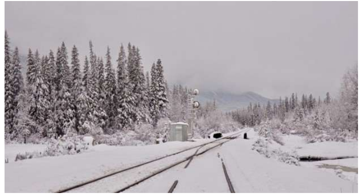
Figure 2. Unheated rail switches accumulate ice and increase the likelihood of unplanned stops or delays.
